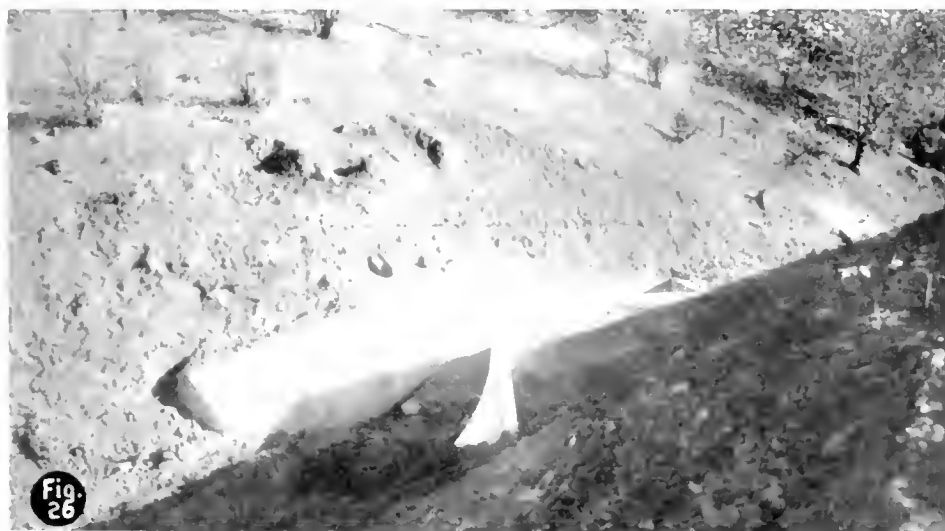
FIG. 26. Open lined training channel to concrete box culvert accelerating stream flow requiring minimum culvert section. Note warped wings
